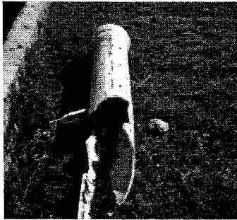
Broken Discharge Pipe
